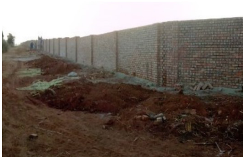
5KM BOUNDARY WALL CONSTRUCTION WITH COMMON BRICKS JOINTED BOTH SIDES
