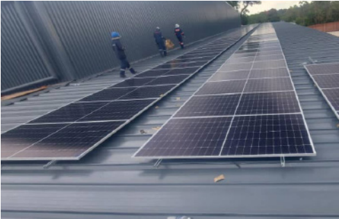
67.2Kwp SOLAR SYSTEM ARRAY FOR A 50KW SOLAR SYSTEM - ELECTROSALES CARDINALS BRANCH
