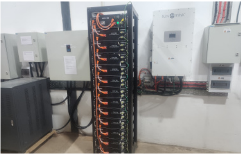
50KW H.V. SOLAR SYSTEM WITH A 62KWH BATTERY BANK - ELECTROSALES CARDINALS BRANCH
