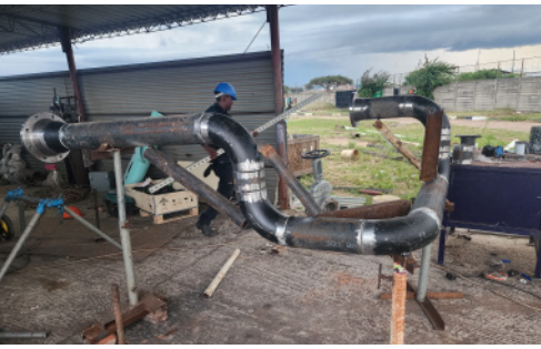
PIPE WORKS FOR A FUEL LINE
