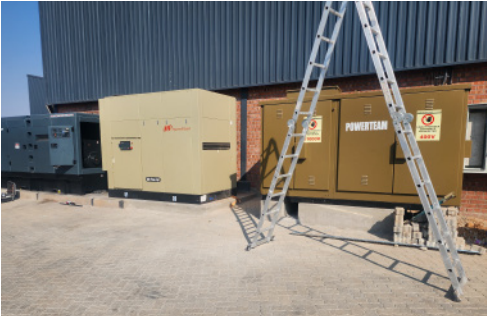
VSD FREE OIL COMPRESSOR AND MINIATURE SUB-STATION - SWAN VALLEY INTERNATIONAL
