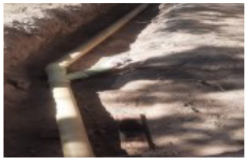
DRAIN LAYING FOR ZELA MAIN SEPTIC TANK
