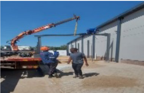
5 TONNE TRUCK AND 15 TONNE SELF LIFTING CRANE
