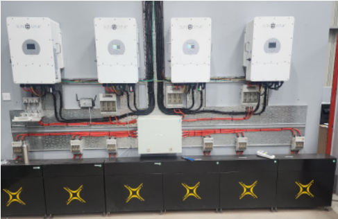
48KW SOLAR SYSTEM WITH A 85.8KWH BATTERY BANK - ELECTROSALES POMONA BUILDERS
