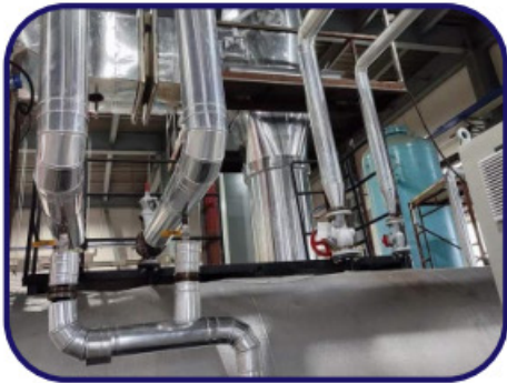
Sandblasting, Lagging & Cladding of plant
