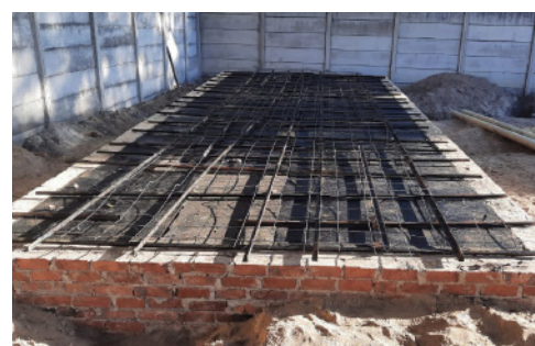
SEPTIC TANK TOP SLAB PREPARATION AT ZELA
