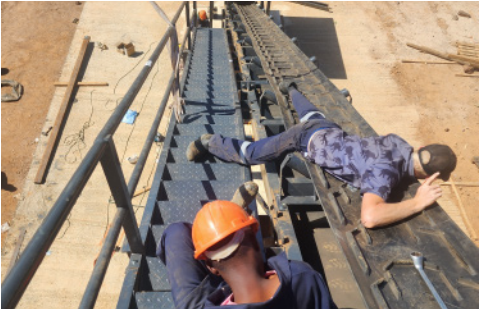
CONEYER ERECTION FOR A CONCRETE BATCHING PLANT - GEO POMONA
